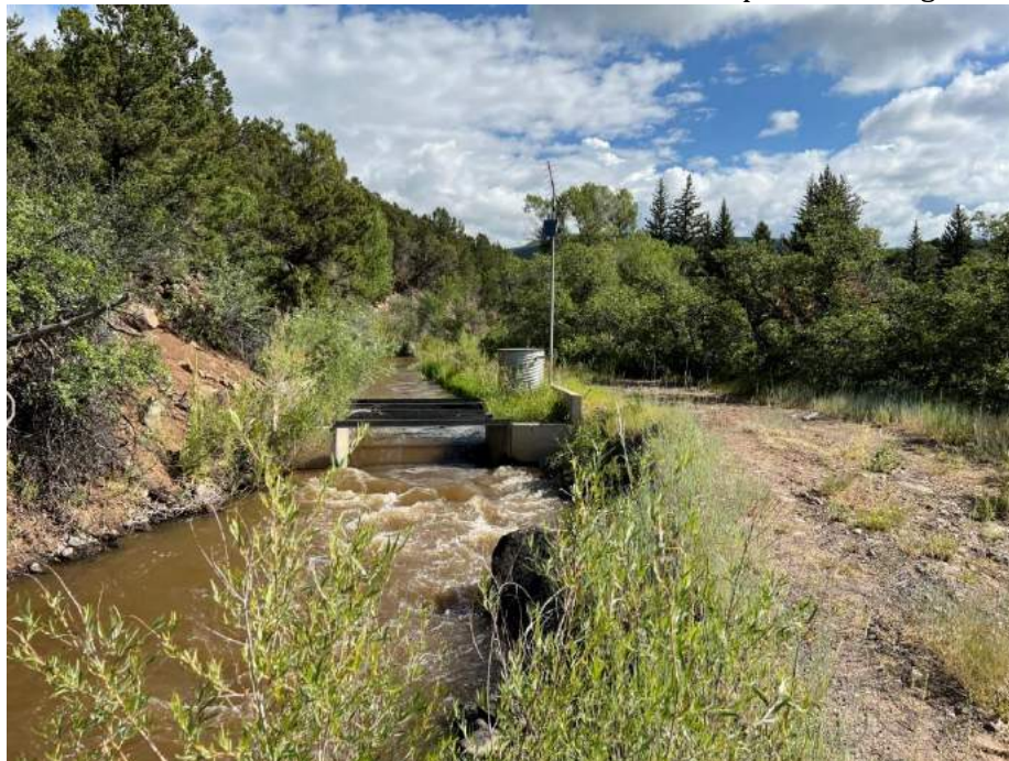
FIGURE 2: OVERLAND 8-FT PARSHALL FLUME WITH TELEMTERY
